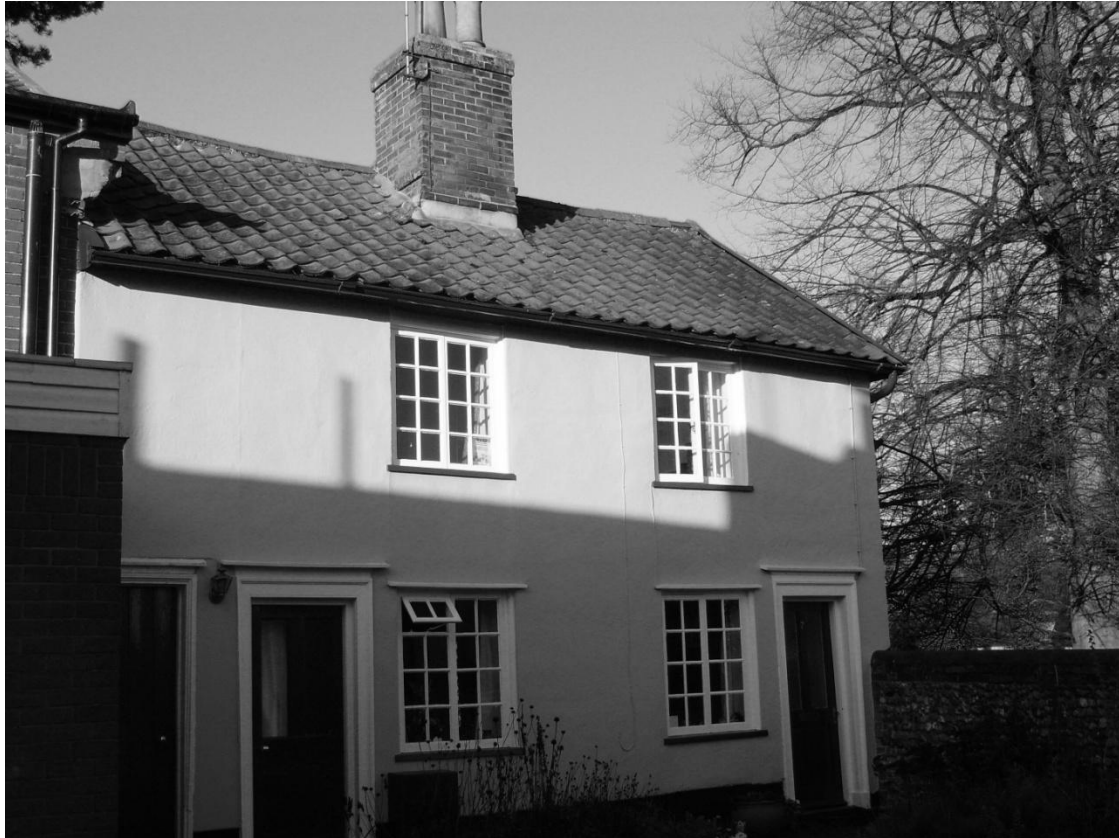
Figure 3: A row of lime-rendered traditional clay-lump cottages in the centre of Diss.
